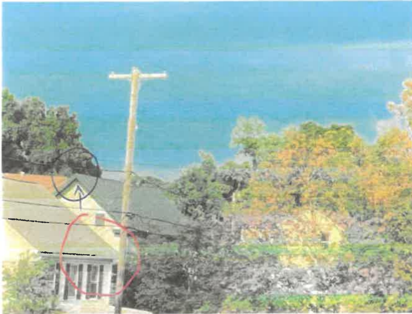
This shows the relatively steep angle of my metal roof. This is the south-facing side.
