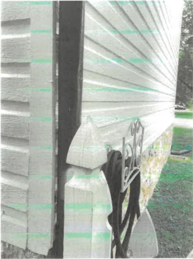
Again, northwest corner, next to back roof downspout. No damage here.
