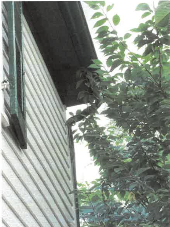
This is the downspout and underside of the existing 6" gutter on the north facing side of the roof to compare how it looks from the ground, compared to the 4" gutter in the front.
